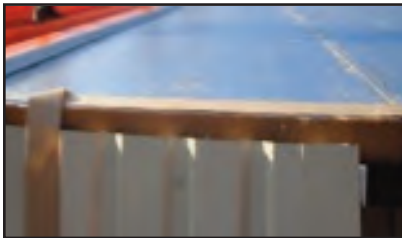
THERMAX™ Insulation with WEATHERMATE™ Flashing Applied
