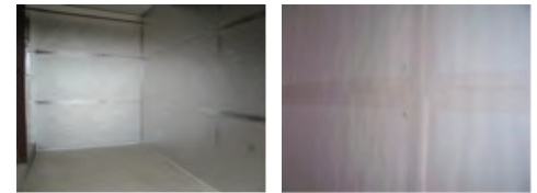
Interior Air Sealing with Tape
