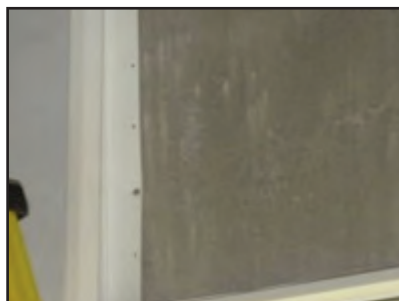
PVC attached to tilt-up wall
